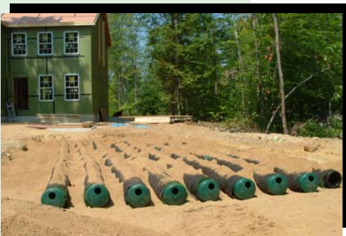
Enviro-Septic® Installation at LEED Certified Home
